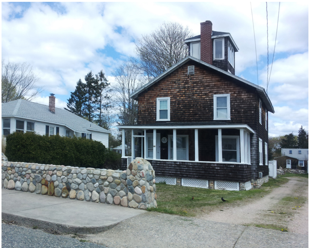
An example of a typical Misquamicut house that has not been significantly damaged in a storm.
