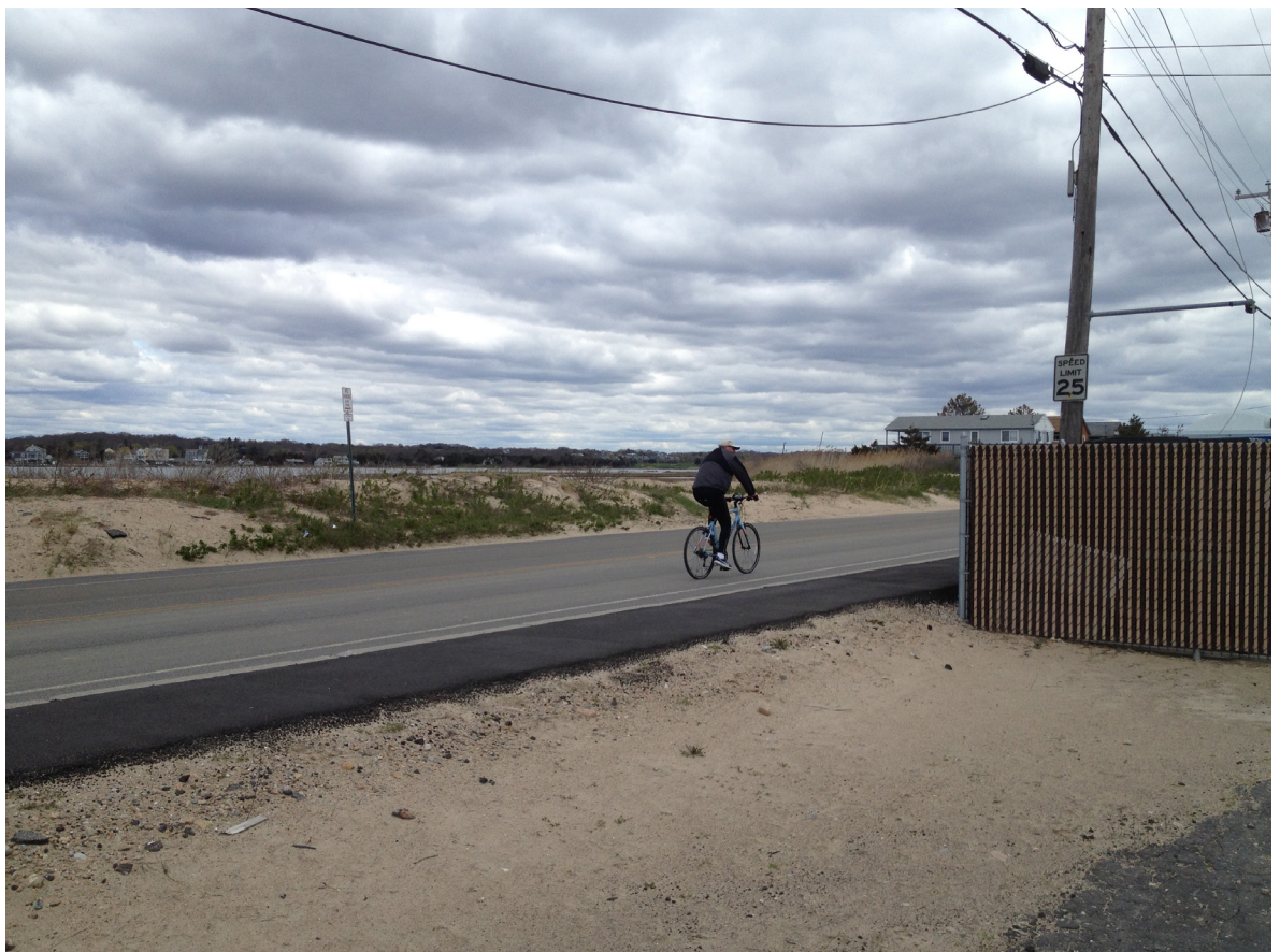
Atlantic Ave. acts as the main thoroughfare in Misquamicut's business district, however it lacks infrastructure to support safe walking or biking.
