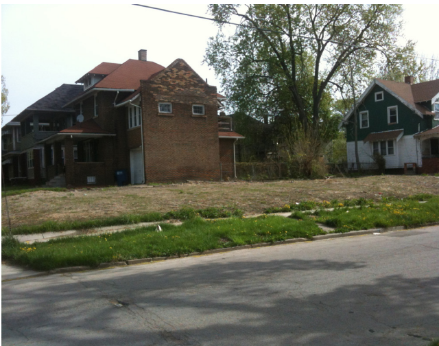
Above: Demolition site with grading towards street and storm drain, resulting in increase stormwater runoff To Right: Quality of the Demolition LCLB Policies & Procedures
