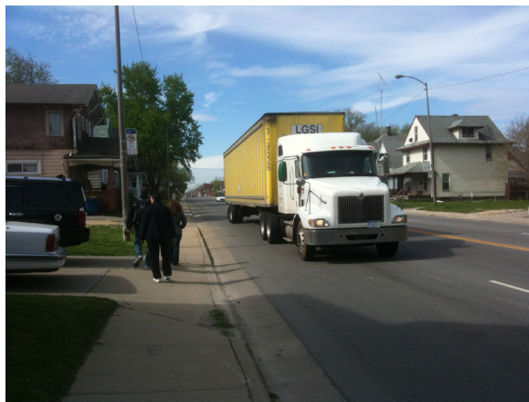
Lack of parkway or planting strip to separate pedestrians from truck traffic on Detroit Avenue
