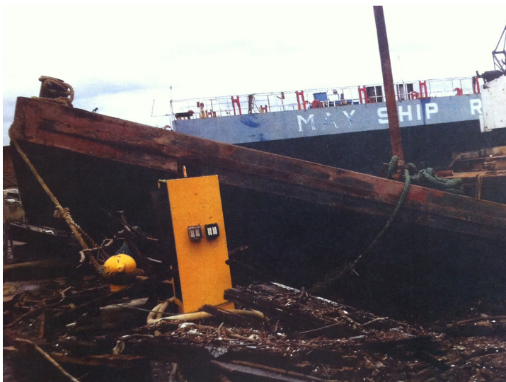
Damage in Richmond Terrace following Hurricane Sandy
