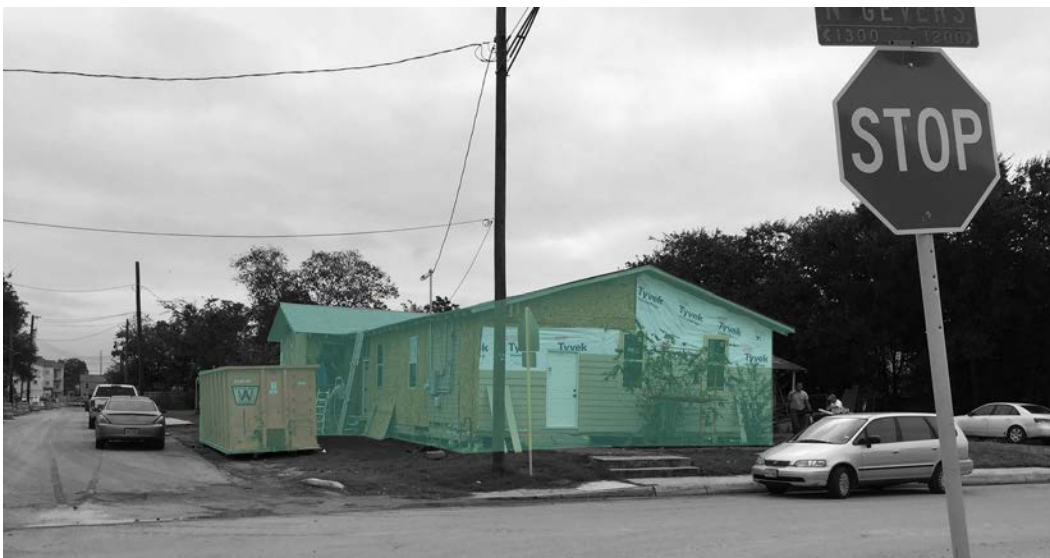
Older home located on North Gevers being rehabbed
