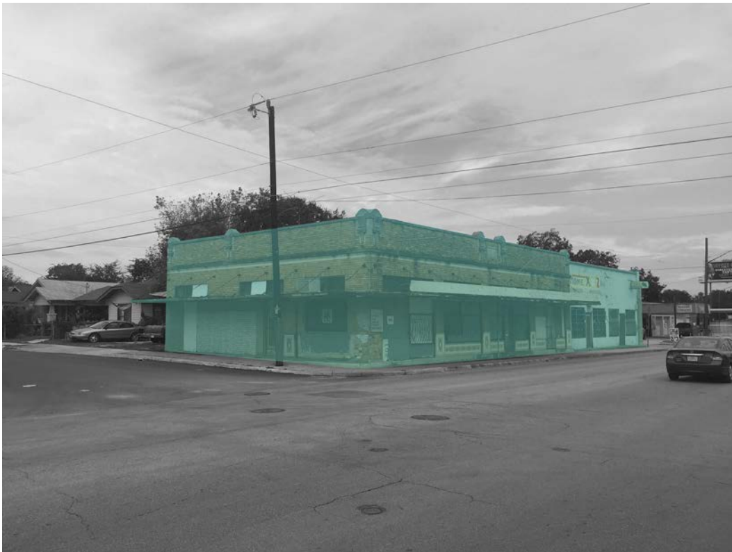
Unoccupied buildings located along New Braunfels commercial corridor
