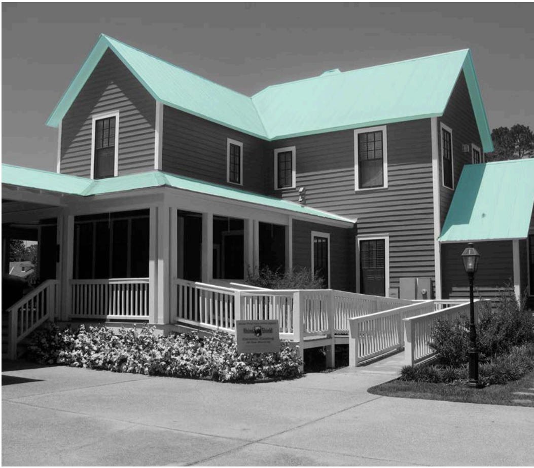
San Antonio Under One Roof program replaces old roof for newer, white, energy efficient roofs
