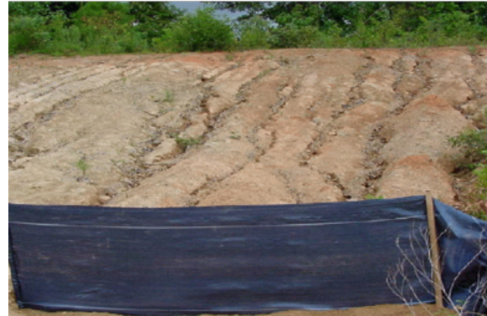
The Silt Fence commonly used for soil and sediment erosion control.
