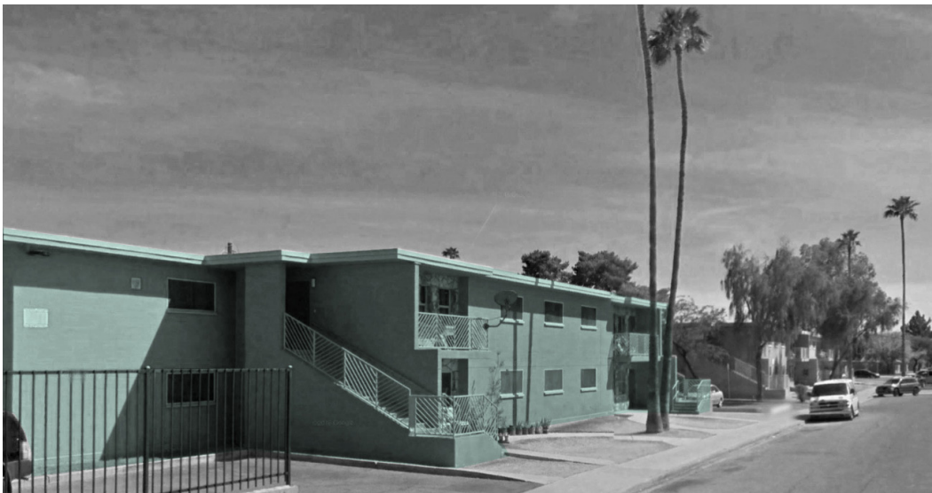
Existing public housing in the District
