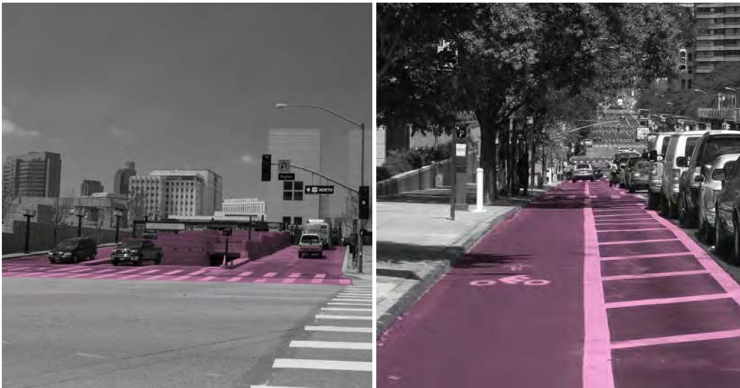
(l) Frequent curb cuts and large garage entrances present conflict points between automobiles and pedestrians and discourage walking (r) A cycle track with buffer in New York City
