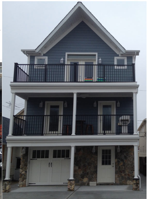
Through the integration of creative facade treatments for non-habitable spaces, a welcoming pedestrian environment can be retained while protecting structures from flooding
