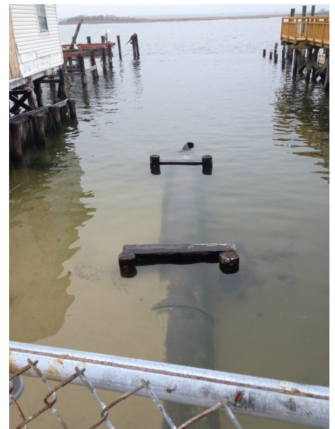
Stormwater outfall into Bay
