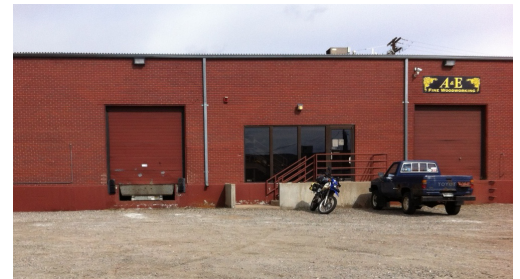
A&E Fine Woodwork- existing warehouse planned for adaptive reuse for artist studios
