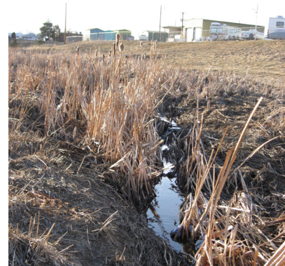
Existing conditions at North Dry Gulch
