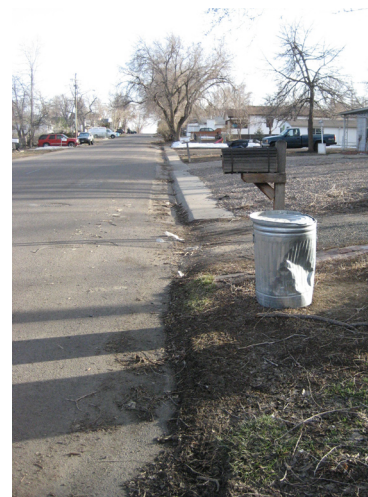
Existing inconsistency in sidewalk network
