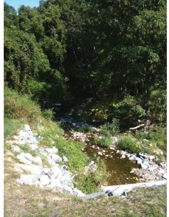
Creek within the assessment area flowing into a street culvert
