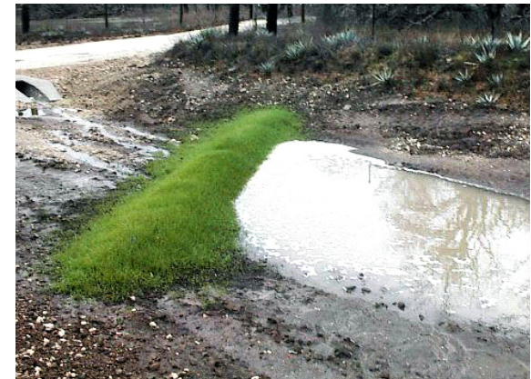
A dike of compost that is applied perpendicular to runoff
