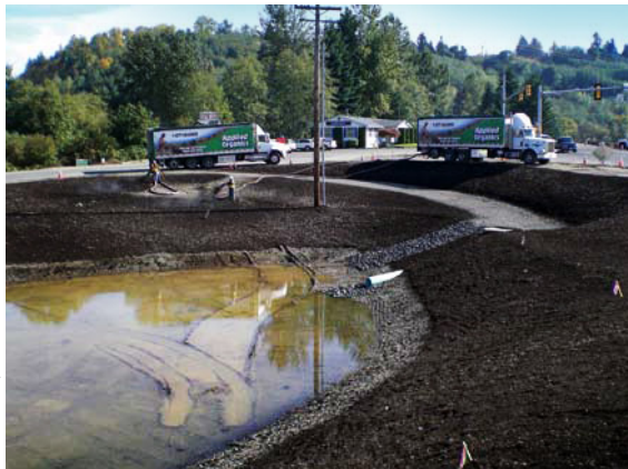
A loose layer of compost applied to the soil in disturbed areas
