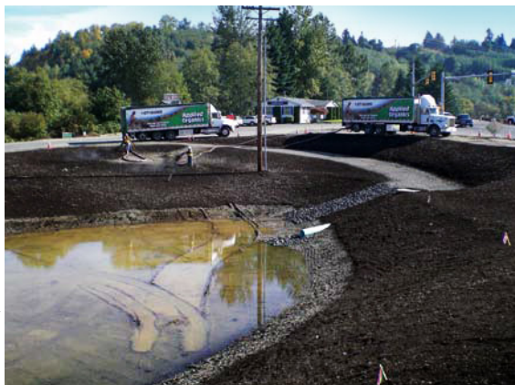
A loose layer of compost applied to the soil in disturbed areas
