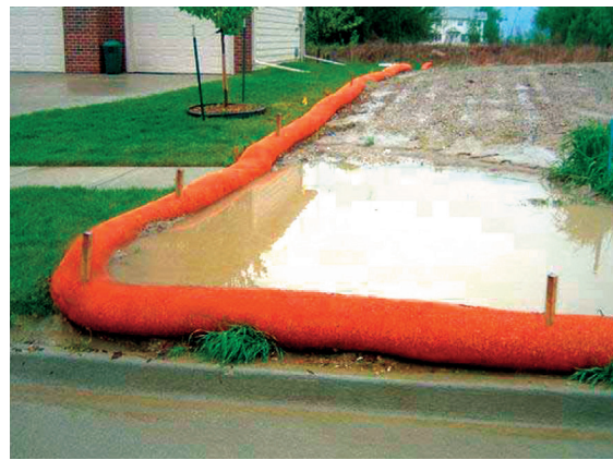
A tube filled with compost placed perpendicular to runoff
