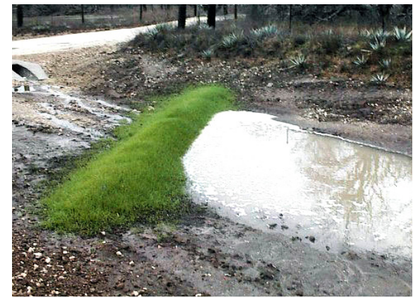
A dike of compost that is applied perpendicular to runoff
