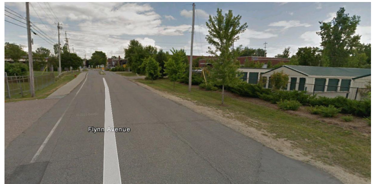
Existing conditions on Flynn Avenue with incomplete sidewalk network
